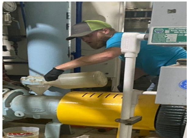
*Pictured right, Wesley Ayers (New employee), slowly fills the bearing housing with oil on the permeate pump.
