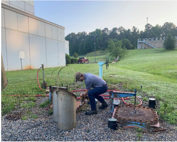
*Pictured left, Clay Stuart tightens the bolts covering the screen chamber.
